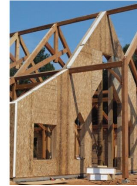
Option 2 – Insulated Panels (IP) Cat 2b
