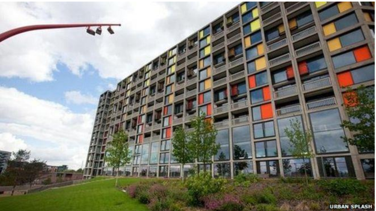
Renovated Park Hill estate, Sheffield. Apartments will be mixed tenure: one third social renting; one third private; one third for sale
