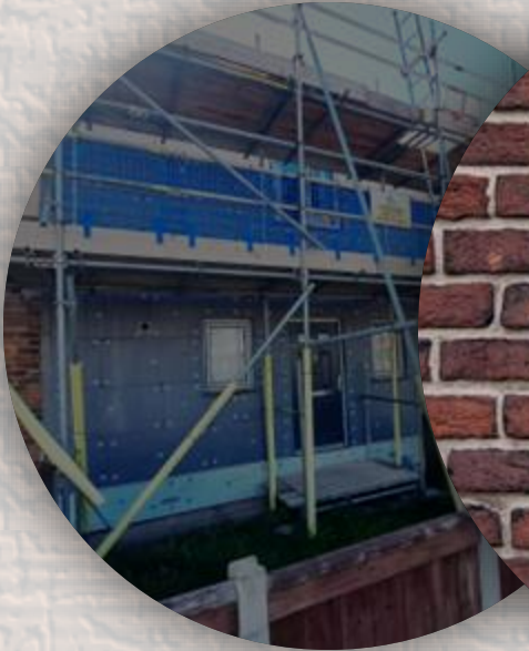
External Wall Insulation and windows/doors
