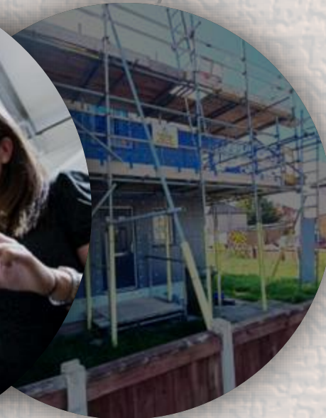
External Wall Insulation and windows/doors
